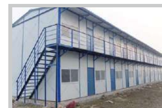
Temporary construction site sewage
