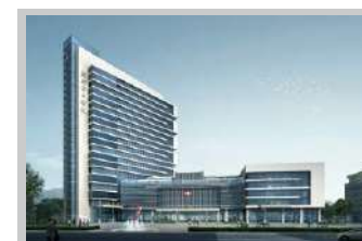
Hospital sewage treatment
