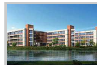
School domes c sewage treatment
